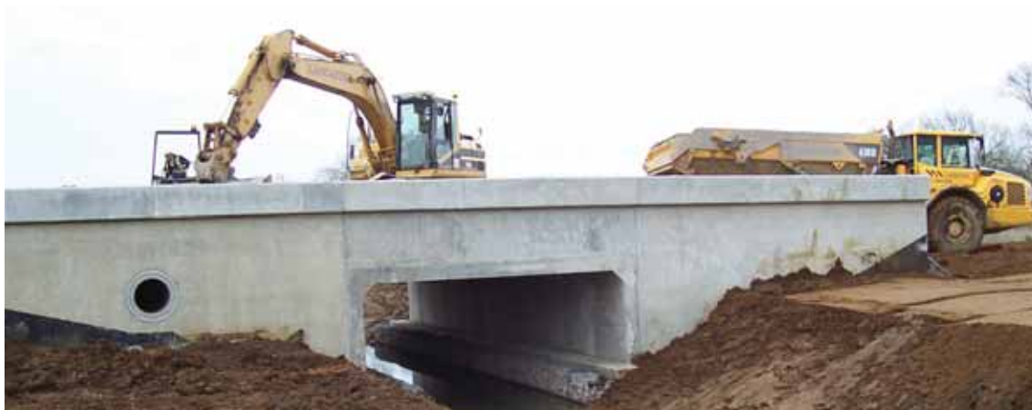
■ Construction of the by-pass over a water way with built in wildlife route
