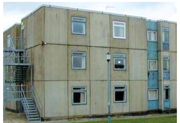
■ Obsolete 1970s concrete barracks
