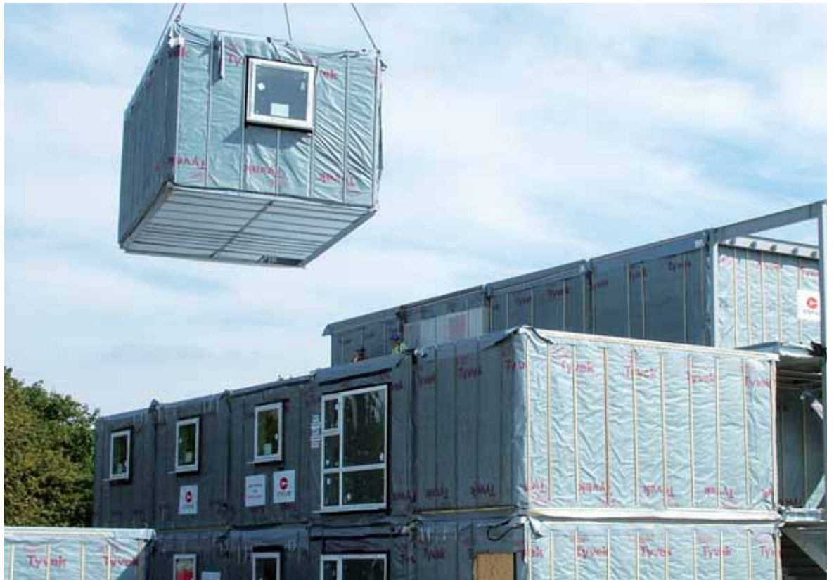
■ on-site construction of modular building
