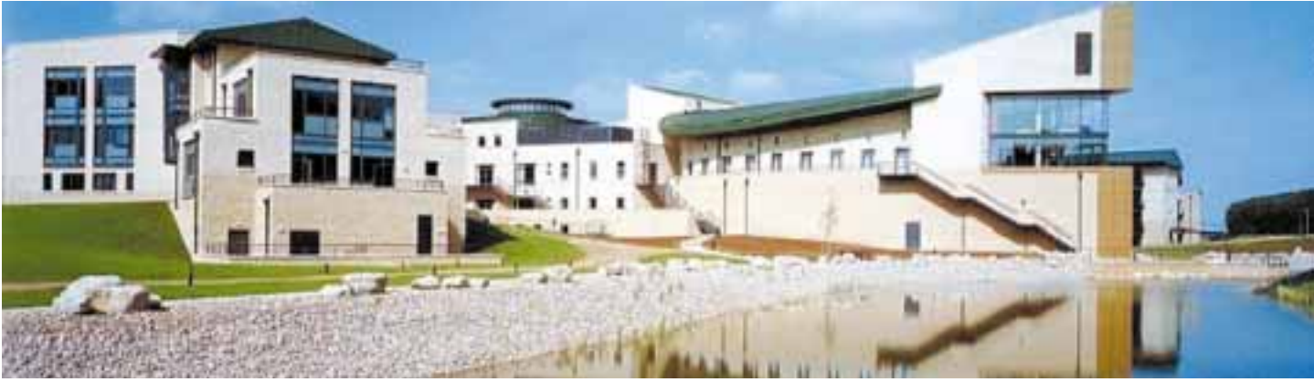
Joint Services Combined Staff College, Swindon
